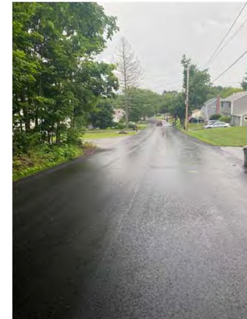
Erlin Road (Mill & Overlay)
