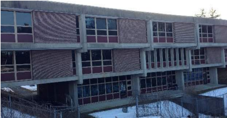
Parker School: Concrete framed with load bearing interior and exterior walls. Constructed in 1965 with a renovation in 2006
