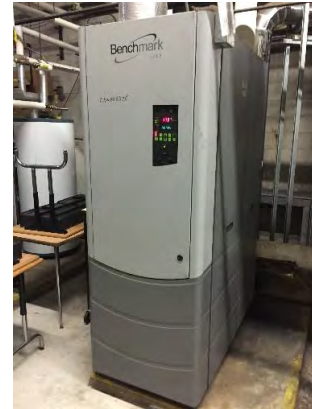
Image 1 – Hot Water Boilers
