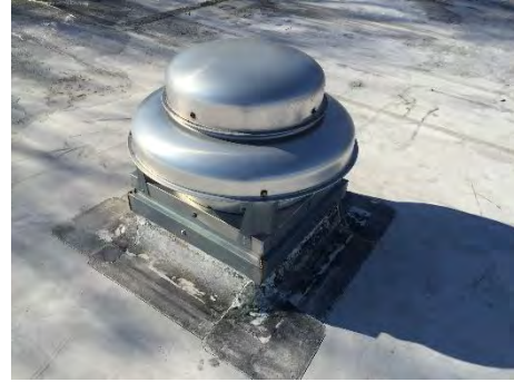
Image 15 – Roof Mounted Exhaust Fan
