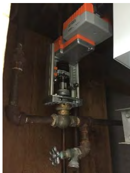
Image 8 – Uninsulated AHU Piping
