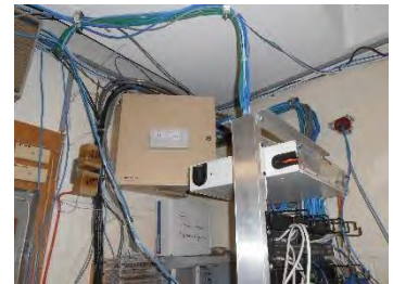
Image 31 – Intrusion System Control Panel
