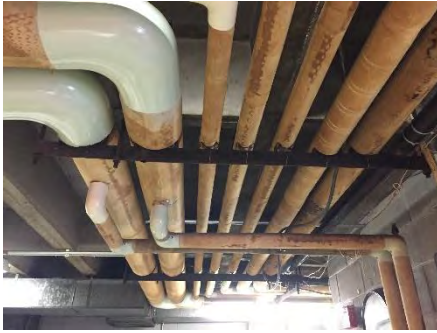
Image 5 – Existing Hot Water Piping
