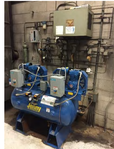
Image 20 – Pneumatic Control System
