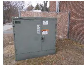
Image 2 – Pad Mount Transformer
