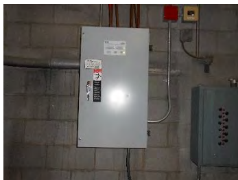
Image 17 – Automatic Transfer Switch
