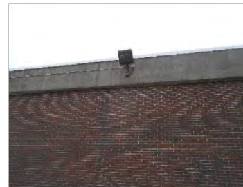
Image 13 – Building Mounted LED
