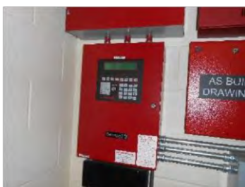
Image 18 – Fire Alarm Control Panel
