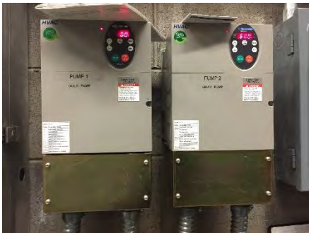
Image 6 – Hot Water Pump VFD Drives
