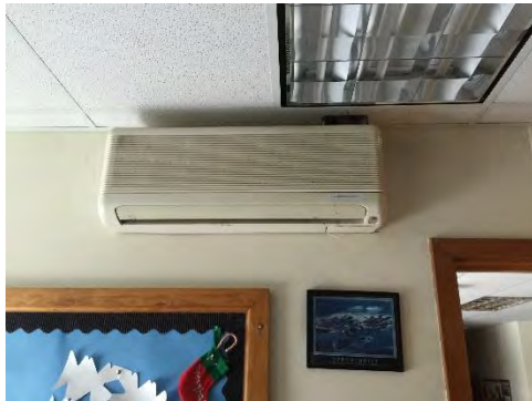
Image 6 – Admin Area Ductless Heat Pump
