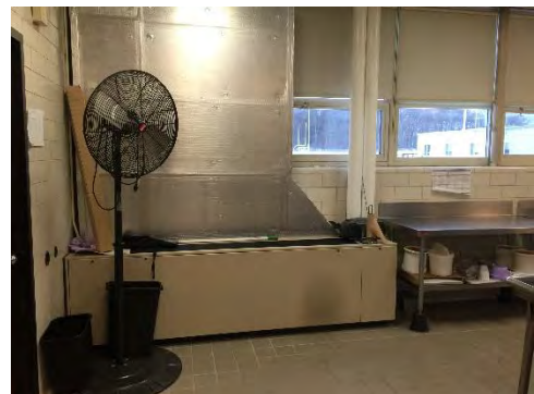
Image 12– Kitchen Unit Ventilator
