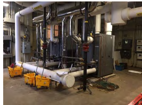
Image 2 - Condensing Boilers (Rear)
