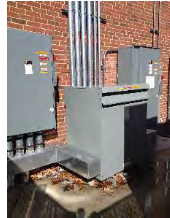
Image 19 –Exterior 300 kVA Step-Down Transformer & Disconnect Switches
