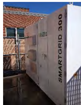
Image 18 – 300 Kw Exterior Inverter
