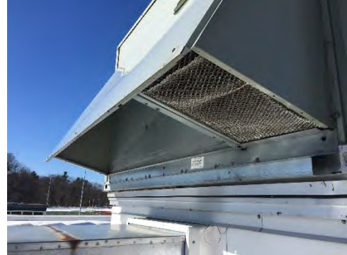
Image 9 – Missing Moisture Elimination Screen on Library RTU
