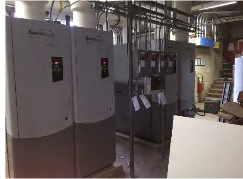
Image 1 - Condensing Boilers
