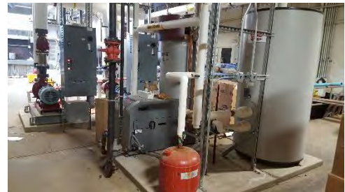
Image 137 – Gas Fired Water Heater & Tank
