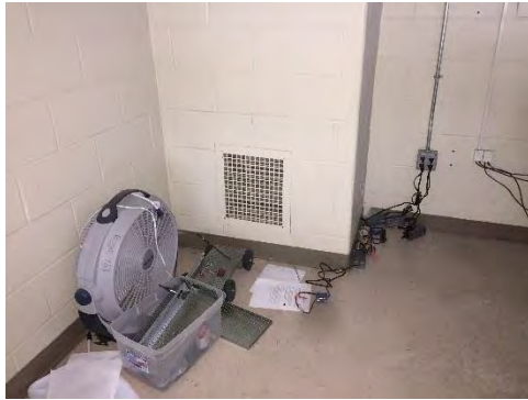
Image 5 – Typical Low Wall Exhaust Grille
