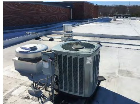
Image 18– Roof Mounted Condensing Unit & Fans
