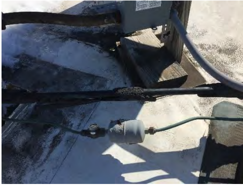
Image 13 – Deteriorated Refrigerant Piping Insulation
