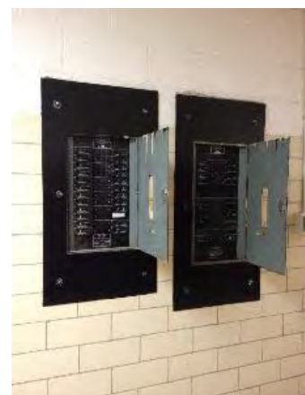
Image 3 – Flush FPE Panels in Corridor
