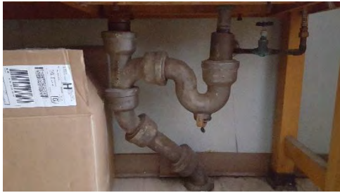
Image 19 – Cast Iron Sanitary Piping
