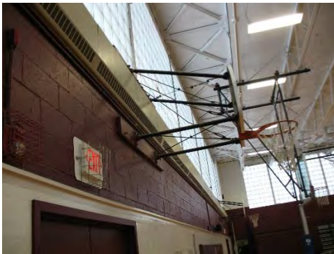
Image 15– Slopetop Radiation at Gym Clerestory
