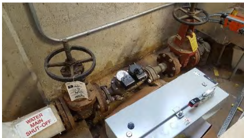
Image 17 – Domestic Water Service & Meter
