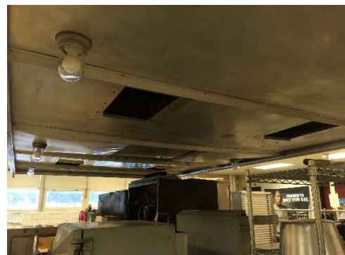
Image 11– Slide Gates Inside Kitchen Hood
