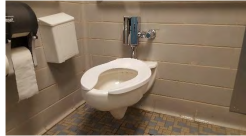
Image 1 – Wall Hung Water Closet
