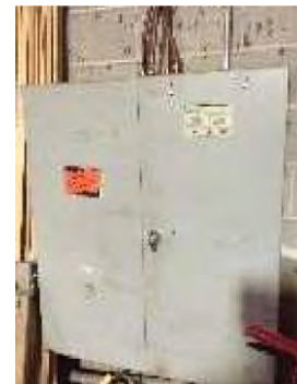
Image 23 — Automatic Transfer Switch
