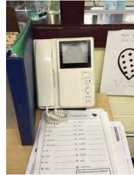
Image 48 – Intercom Master Station
