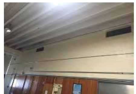
Image 12 – Cafeteria Supply Diffusers
