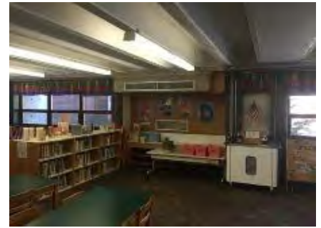
Image 9 – Library Unit Ventilator
