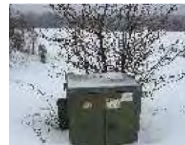
Image 2 — Pad Mount Transformer
