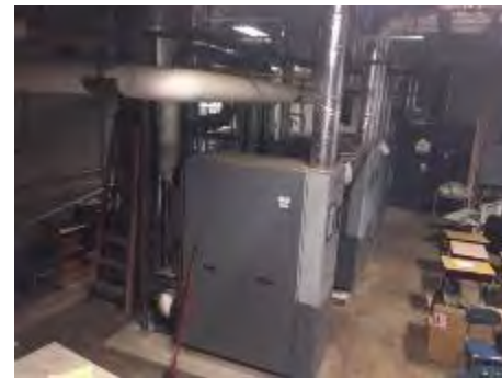
Image 1 – Hot Water Boilers
