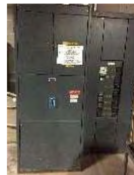
Image 3 — Main Switchgear
