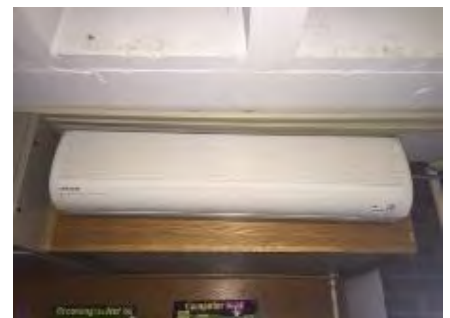
Image 11 – Ductless AC Unit (Technology Class Room)
