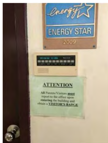
Image 47 – Intrusion Keypad
