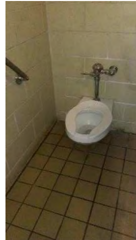
Image 1 — Wall Hung Water Closet
