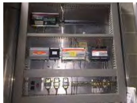
Image 23 – ATC Controls and Control Panel
