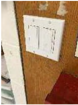
Image 17—Typ. Low Voltage Classroom Switches
