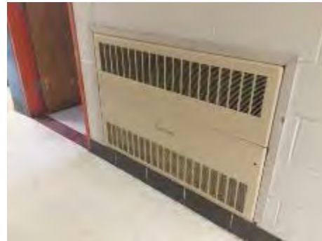
Image 21 – Corridor Hot Water Unit Heater
