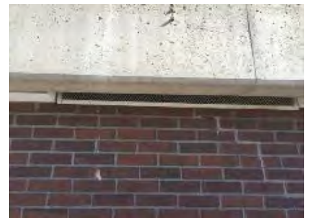
Image 10 – Unit Ventilator Louver
