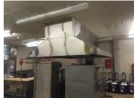
Image 14 – Kitchen Exhaust Hood
