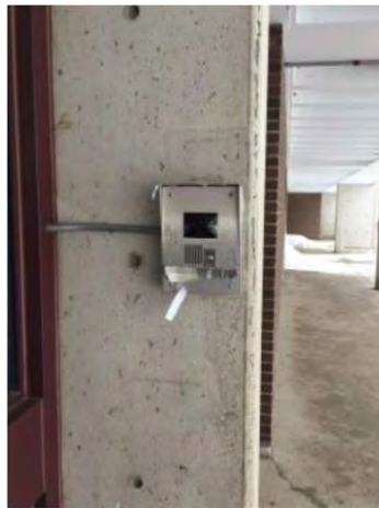
Image 46 – AI Phone Intercom at Main Entrance
