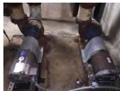
Image 4 – Hot Water Pumps
