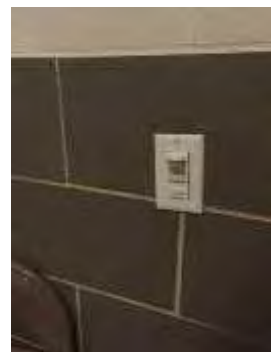
Image 16 – Occupancy Sensor Switch
