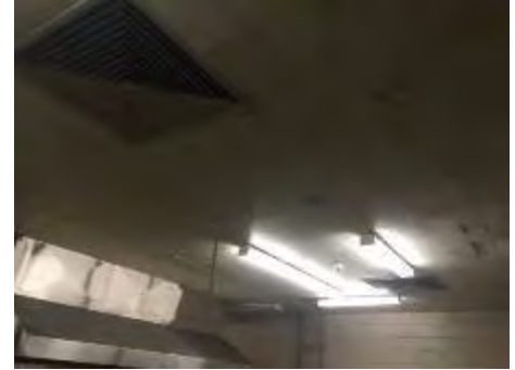
Image 13 – Kitchen Make-up Air Supply Diffusers
