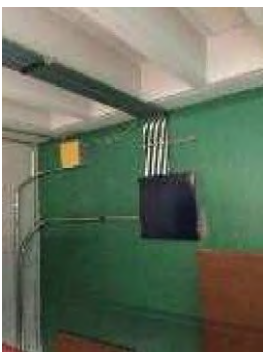
Image 8— New Branch Circuit Install
