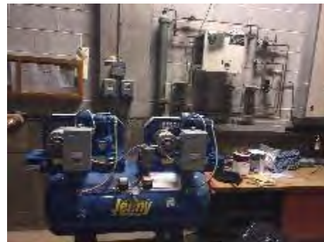
Image 22 – Pneumatic Compressor
