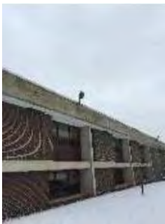
Image 19— Bldg. Mounted LED Flood
