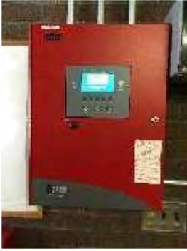
Image 25— Fire Alarm Control Panel
