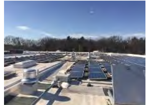
Image 19 – Roof Exhaust Air Fans
