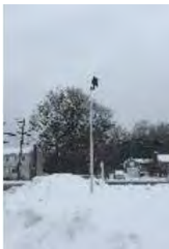
Image 18— Pole Mounted LED Flood
