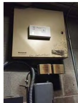
Image 49 – Intrusion System Panel
