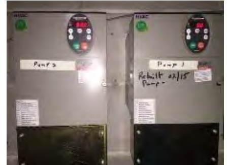
Image 5 – Hot Water Pump VFD Drives
