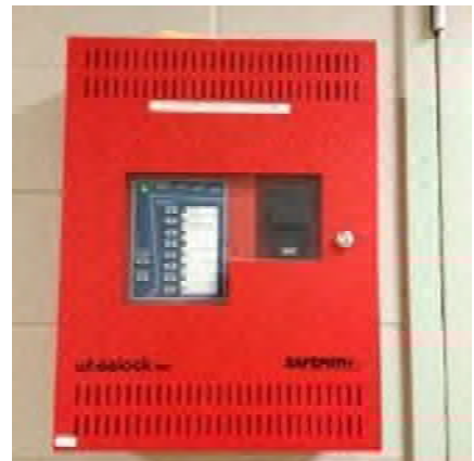
Figure 23 – Voice Evac Panel in Auditorium
