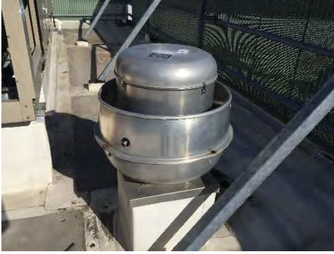
Figure 11 – Roof Exhaust Fan
