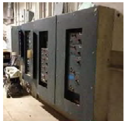
Figure 6 – Motor Control Center
