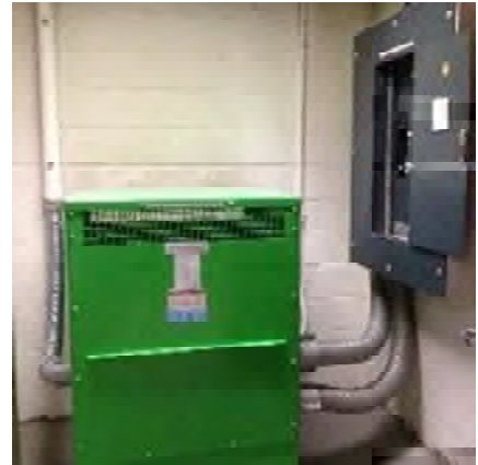
Figure 4 – New Transformer
