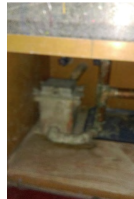
Figure 8 – Plaster Trap
