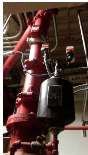
Figure 2 – Dry alarm Check
