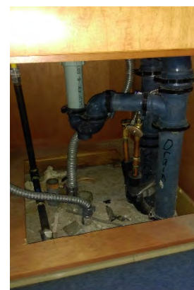
Figure 9 – Science Sink Piping
