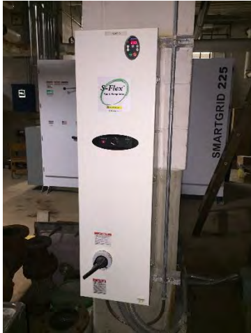
Figure 4 – Pump VFD Drive
