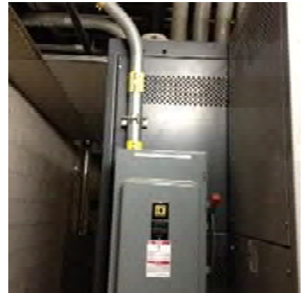
Figure 7 – Tapped Disconnected Switch for ATS 2
