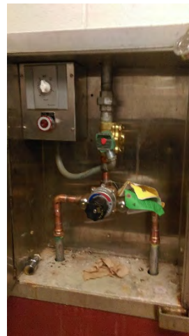
Figure 12 – Mixing Valve
