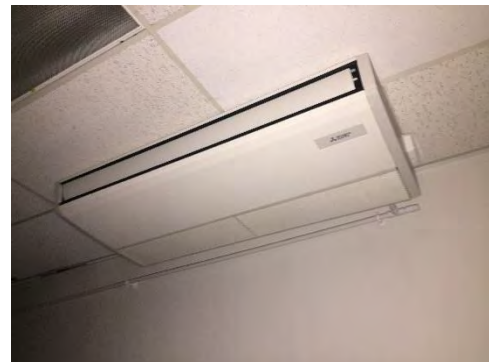
Figure 9 – Ductless AC Unit
