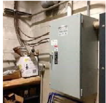
Figure 19 – ATS 1 in Boiler room
