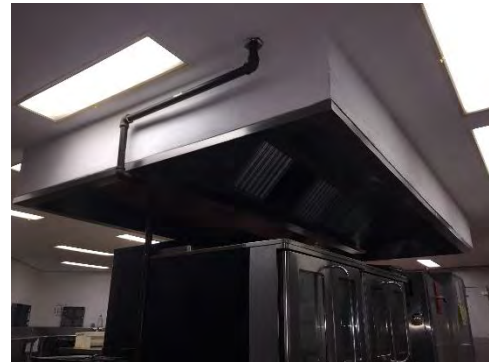
Figure 8 – Kitchen Exhaust Hood
