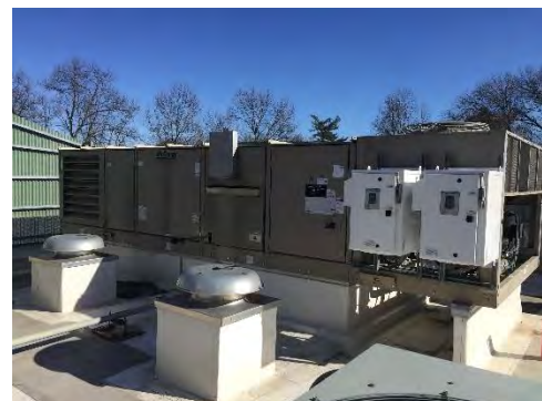
Figure 10 – Rooftop Air Handling Unit
