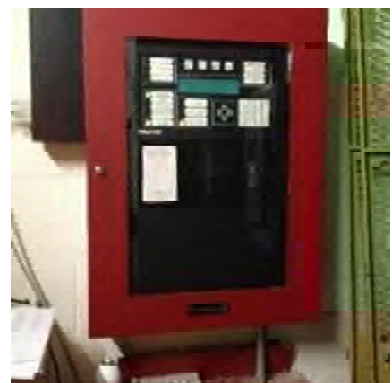
Figure 21 – FACP in Electric Room
