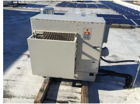
Figure 15 – Ductless AC Unit Condensing Unit
