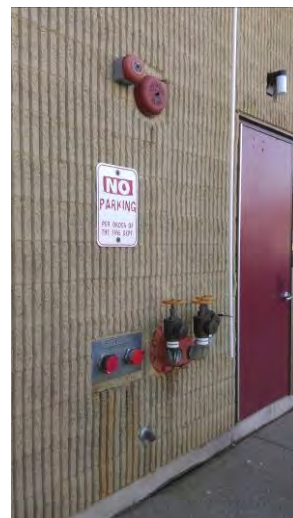
Figure 3 – FDC and Test Header
