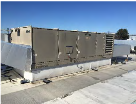
Figure 14 – Rooftop Air Handling Unit
