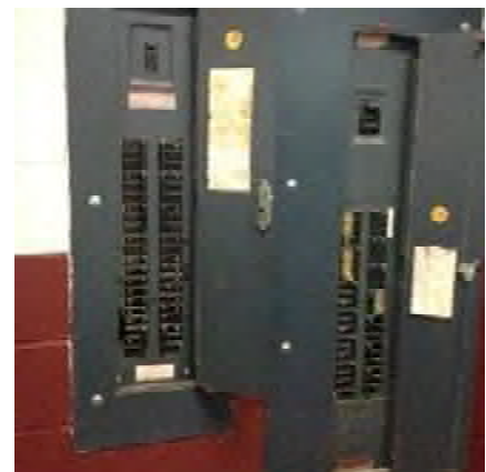
Figure 3 – Typical Original GE panels
