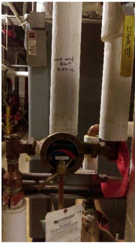
Figure 16 – Mixing Valve
