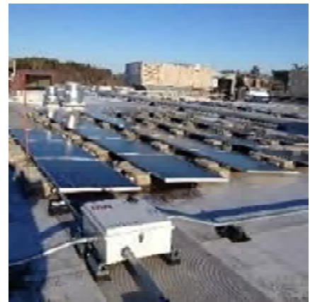
Figure 26 – Roof PV Panels
