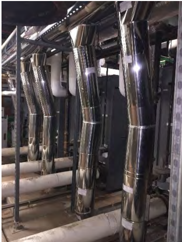
Figure 2 – Boiler Breaching
