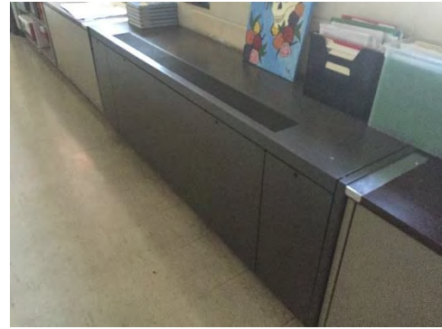
Figure 7 – Classroom Unit Ventilator
