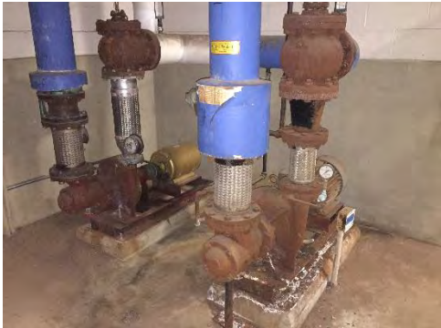
Figure 3 – Hot Water Pumps
