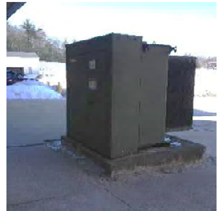
Figure 1 – Pad Mounted Transformer
