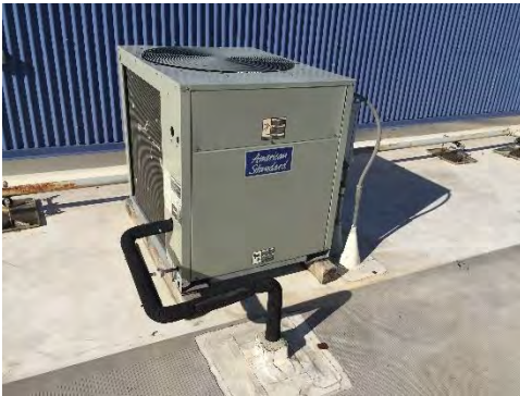
Figure 12 – Air Cooled Condensing Unit
