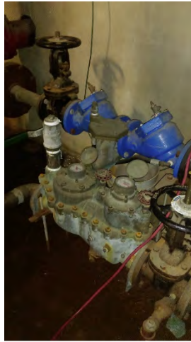
Figure 14– Water Meter
