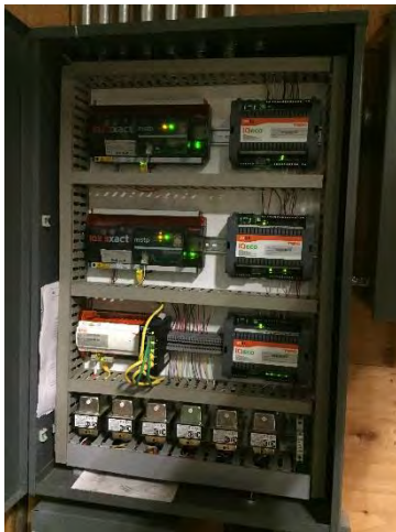
Figure 5 – ATC/DDC Control Panel
