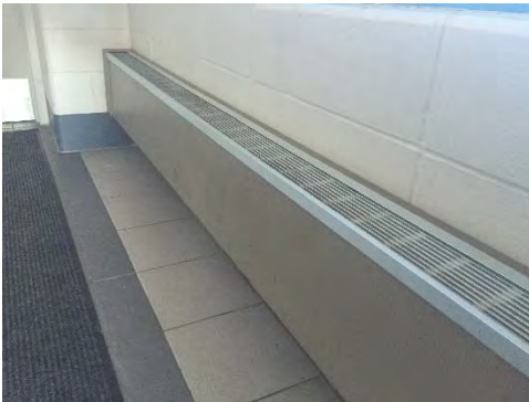
Figure 13 – Fin Tube Radiation
