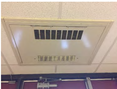
Figure 6 – Entryway Cabinet Unit Heater
