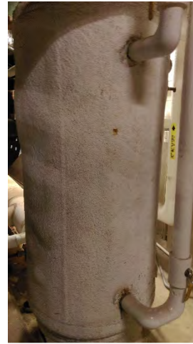
Figure 15 – Domestic Storage Tank
