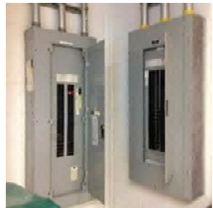
Figure 8 – Newer Surface Panels in Corridor
