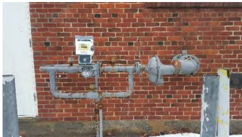
Image 19 – Gas Service & Meters
