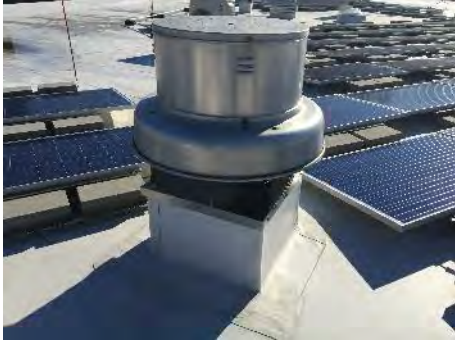
Image 15 – Roof Mounted Exhaust Fan
