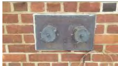
Image 3 – Fire Department Connection
