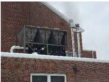
Image 8 – Air Cooled Chiller
