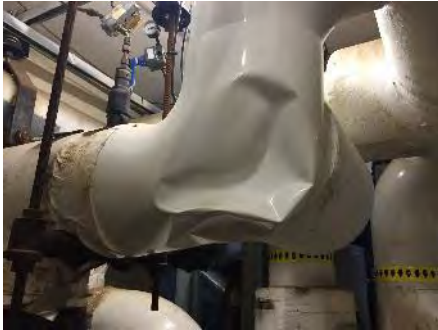
Image 5 – Existing Damaged Piping Insulation
