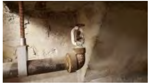
Image 6 – Upright Sprinkler Head
