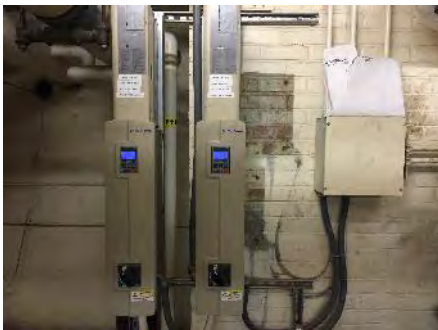
Image 7 – Hot Water Pump VFD Drives
