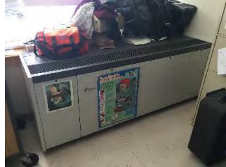
Image 9 – Vertical Unit Ventilator
