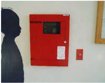
Image 18 – Fire Alarm Control Panel
