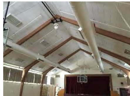
Image 14 – Gym Distribution Ductwork
