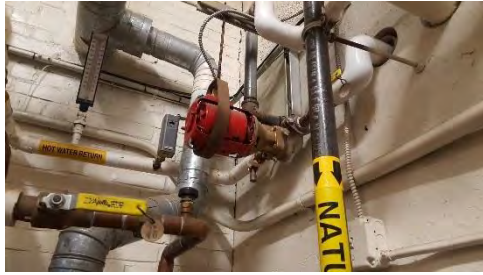
Image 17 – Hot Water Recirculating Pump
