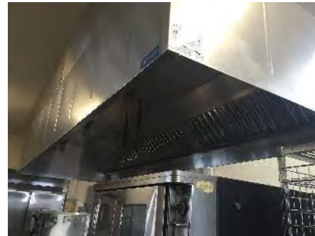
Image 12 – Kitchen Exhaust Hood
