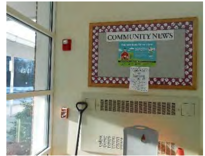
Image 20 – Pull Station & Horn/Strobe
