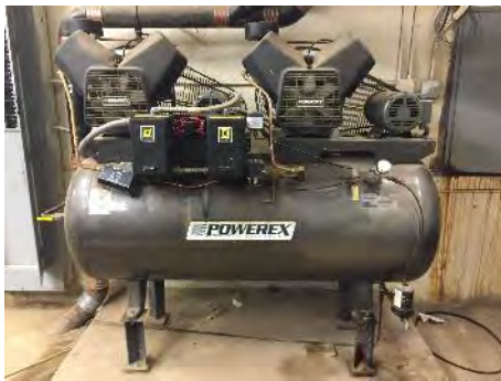
Image 20 – Pneumatic Control System
