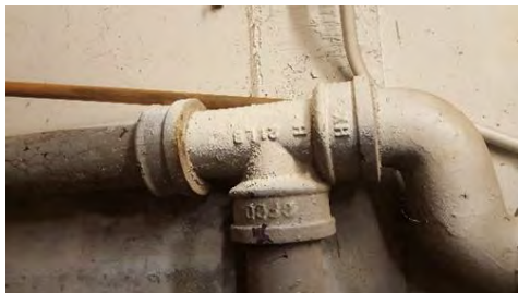
Image 20 – Cast Iron Piping
