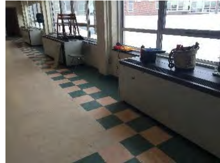
Image 13 – Cafeteria Unit Ventilators
