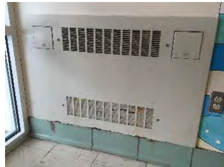
Image 18 – Corridor Unit Heater
