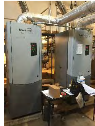
Image 1 – Hot Water Boilers
