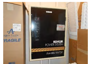
Image 17 – Automatic Transfer Switch
