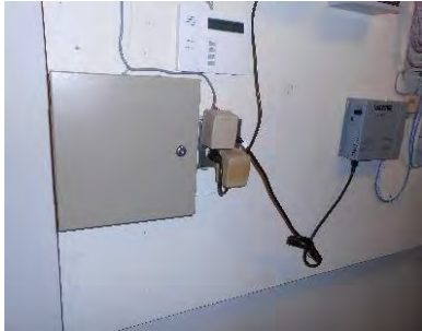
Image 30 – Intrusion System Control Panel & Keypad
