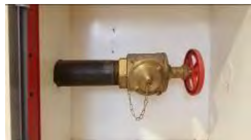
Image 4 – Fire Department Valves
