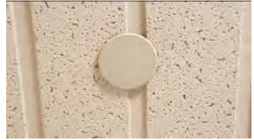
Image 5 – Concealed Sprinkler Head
