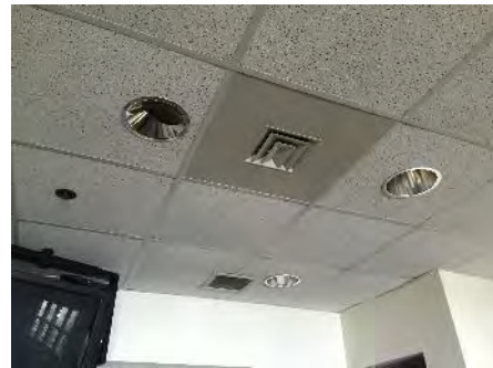
Image 10 – Ceiling Mounted Diffuser
