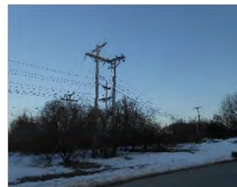
Image 1 – Utility Pole Riser
