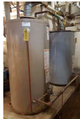
Image 16 – Gas Fired Water Heaters
