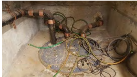
Image 22 – Duplex Sewer Ejector Pit
