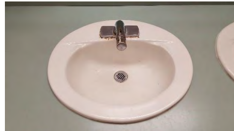
Image 5 – Counter mounted Lavatory
