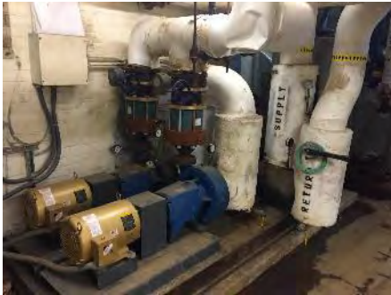
Image 6 – Hot Water Pumps
