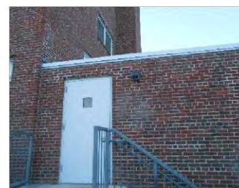
Image 13 – Building Mounted LED Flood
