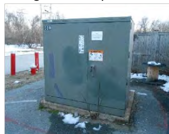
Image 2 – Pad Mount Transformer
