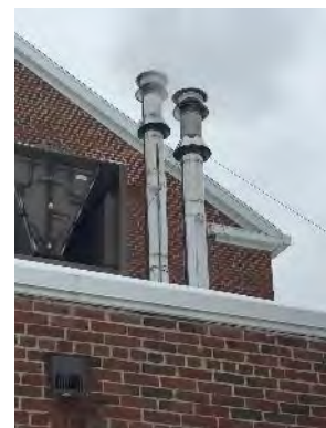
Image 3 – Boiler Flue Vents
