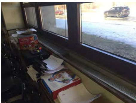
Image 8 – Perimeter Fin Tub Radiation
