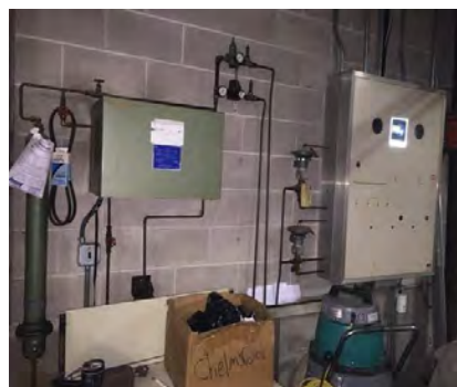
Image 26 – ATC Controls & Control Panel
