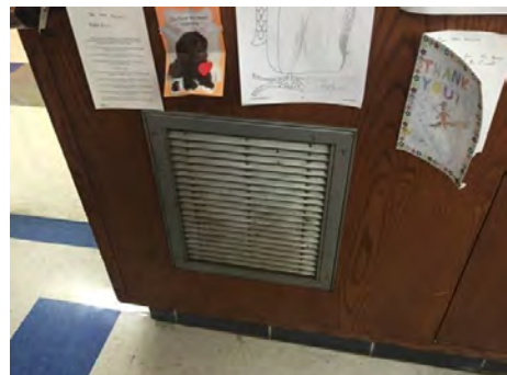
Image 11 – Typical Classroom Exhaust Grille
