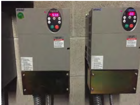
Image 6 – Hot Water Pump VFD Drivers
