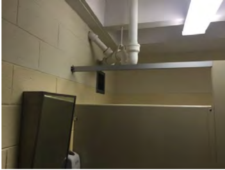
Image 21 – Restroom Exhaust Grille
