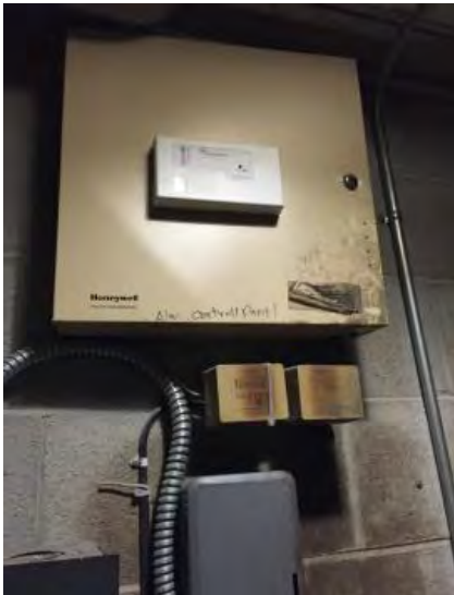
Image 36 – Intrusion System Control Panel
