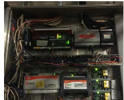
Image 27 – DDC Control Panel
