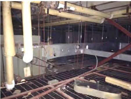
Image 15 – Kitchen Make-up Air Unit
