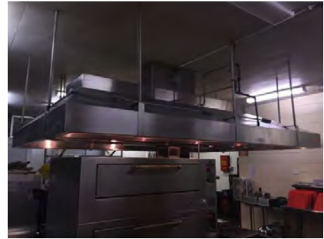
Image 17 – Kitchen Exhaust Hood
