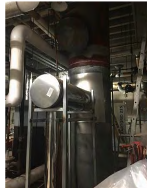
Image 2 – Boiler Flue Vents
