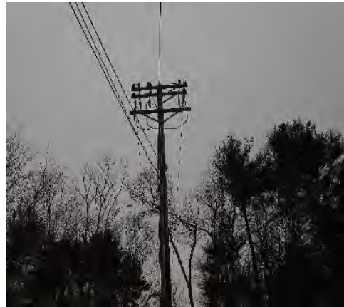
Image 1 – Utility Pole Riser
