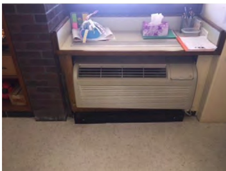
Image 7 – Admin. Office PTAC Unit
