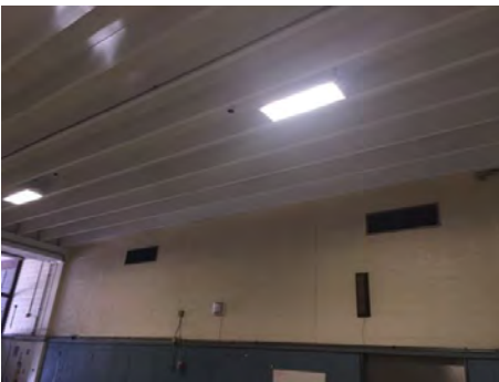
Image 14 – Cafeteria Supply Diffusers
