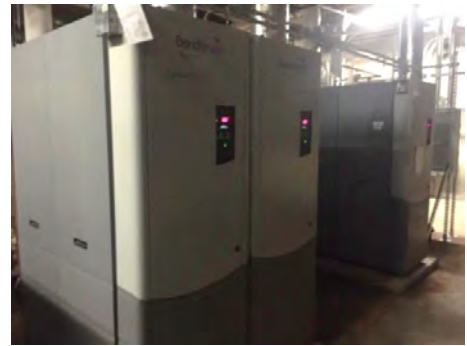
Image 1 – Hot Water Boilers
