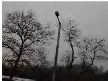
Image 15 – Pole Mounted LED Flood
