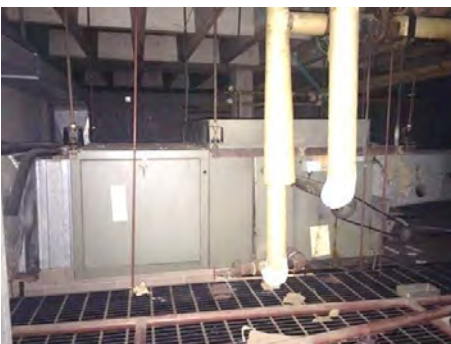
Image 16 – Cafeteria H&V Unit
