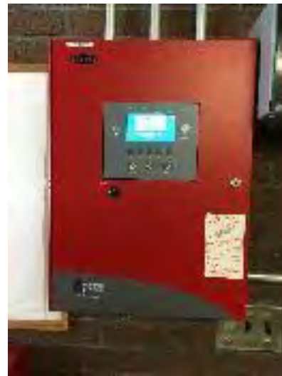
Image 20 – Fire Alarm Control Panel
