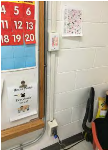
Image30 – A/U Control System
