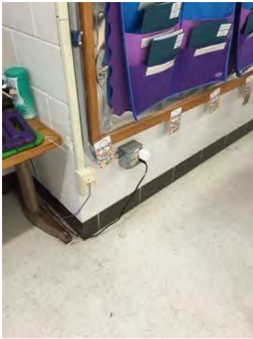
Image 29 – Classroom Data Wiring
