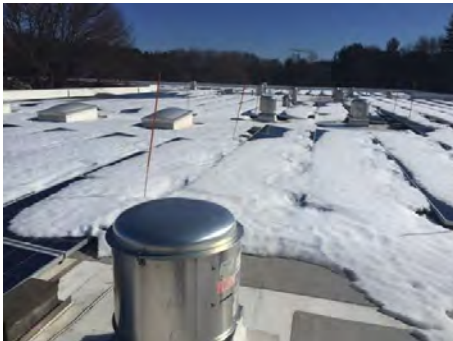
Image 22 – Restroom Exhaust Air Fans
