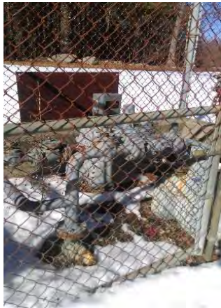
Image 10 – Gas Service and Meter
