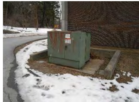
Image 2 – Pad Mount Transformer
