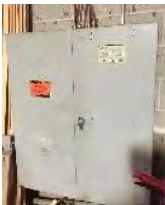
Image 19 Automatic Transfer Switch
