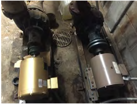
Image 5 – Hot Water Pumps
