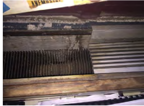
Image 9 – Fin Tube Radiation Heating
