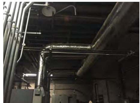
Image 4 – Hot Water Pumps
