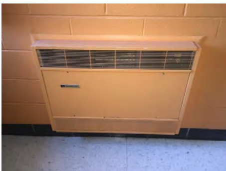
Image 24 – Corridor Hot Water Unit Heater
