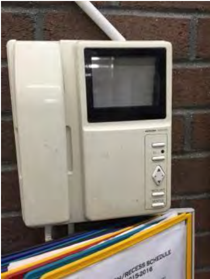
Image 35 – Intercom Master Station
