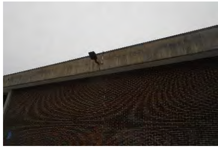
Image 16 – Building Mounted LED
