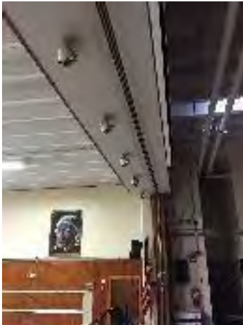
Image 10 – Platform Track Lights
