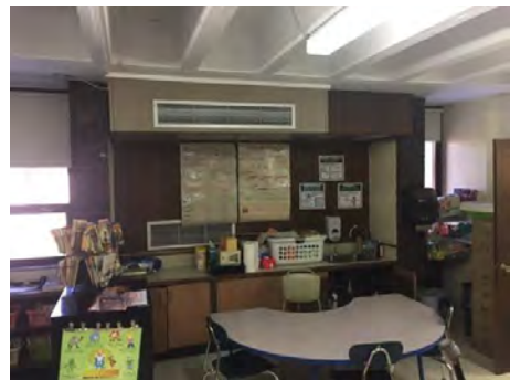
Image 10 – Typical Classroom Unit Ventilator
