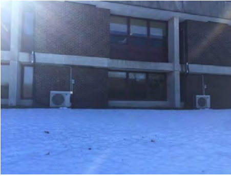
Image 13 – Ductless AC Unit Condensers
