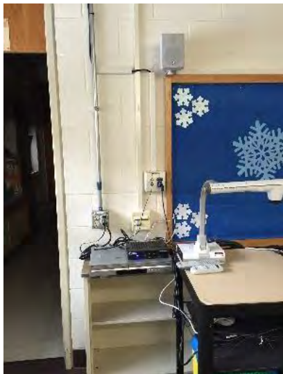
Image 6 – New Branch Circuit Install
