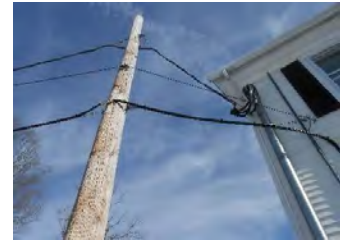
Image 1 – Utility Pole w/ Secondary Service Drop
