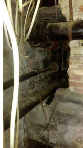
Image 10 – Cast Iron Drainage
