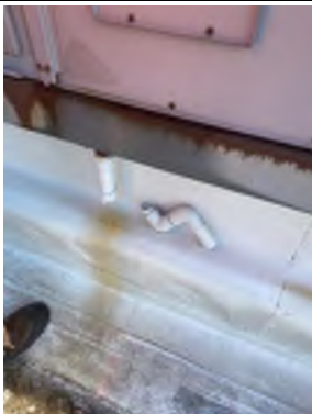
RTU-17 Condensate Trap
