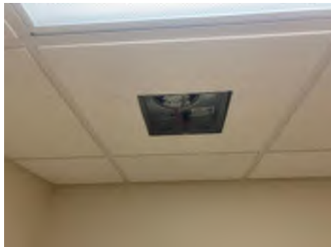
Nurse Restroom - Needs RGD
