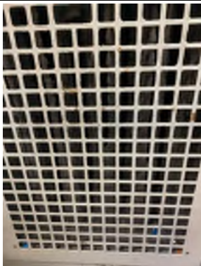
Exhaust RGD's need to be cleaned along with duct
