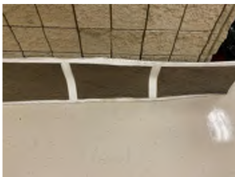
Unit ventilator in room 255 (ceiling mounted unit)
