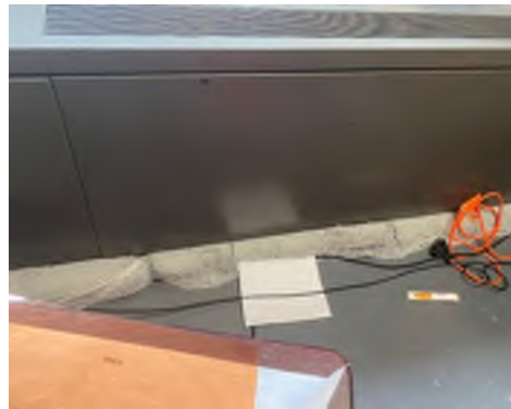
Studio - Foam blocking the return on the unit ventilator
