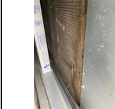
Evaporator coils
