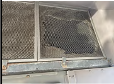
CONDITION OF ECONOMIZER FILTERS
