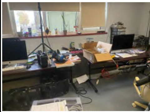
Studio - Unit Ventilator behind everything
