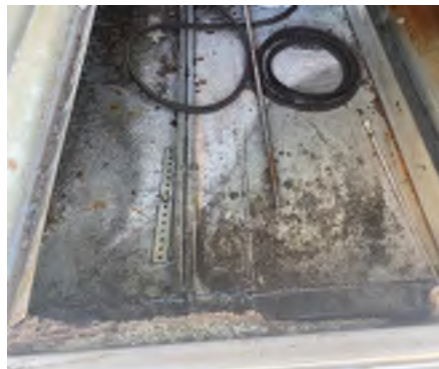
RTU-17 - Water in the unit - not the drain pan
