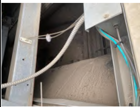
Many of the return ducts - need to be cleaned
