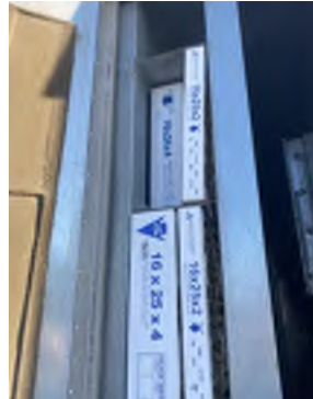
RTU-8 Incorrect filters
