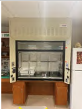
Fume hoods - in rooms 111 & 117
