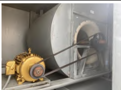
RTU-11 - inner belt is very loose - a video can be provided if needed.
