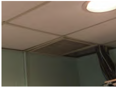
Studio - Foam blocking the return on the unit ventilator
