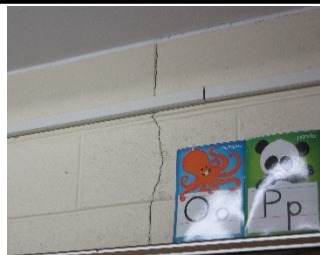
4. Cracks in walls
