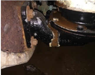
7. Condenser Pump leak
