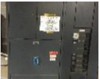
8. Ungrounded switchgear
