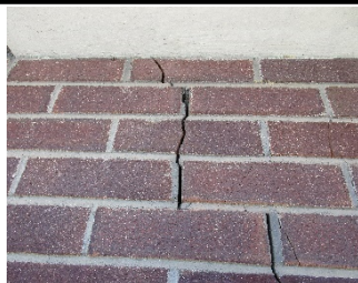
3. Cracks in walls
