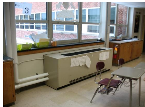
Image 20– Typical Classroom Unit
