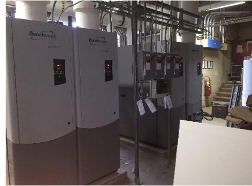
Image 1 - Condensing Boilers
