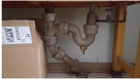
Image 19 – Cast Iron Sanitary Piping
