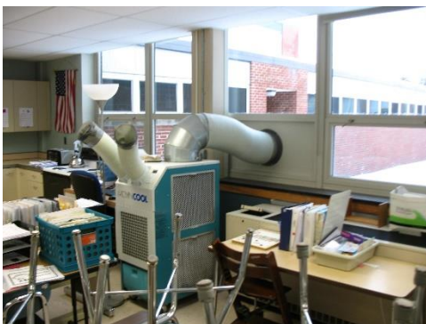
Image 16– Portable Air Conditioner
