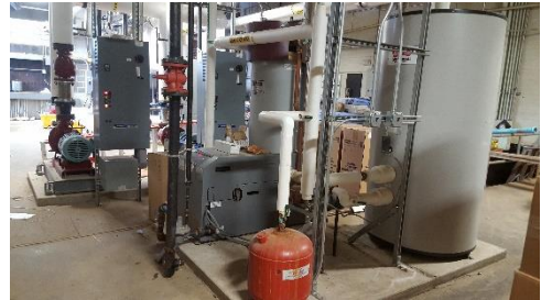
Image 137 – Gas Fired Water Heater & Tank
