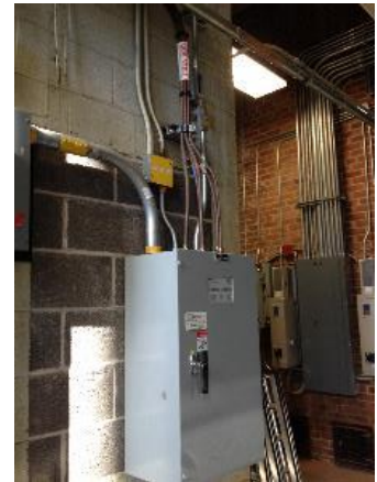
Image 14 – ATS 1 in Boiler Room
