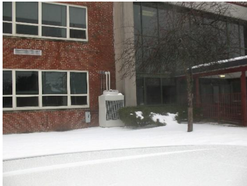
Image 7 – Admin Area Condensing Unit
