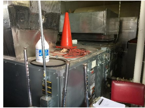
Image 17 – Auditorium Air Handler
