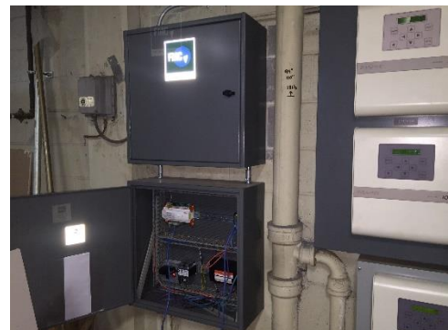
Image 4 - DDC Control Panel
