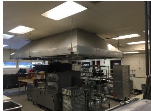
Image 10– Canopy Kitchen Hood
