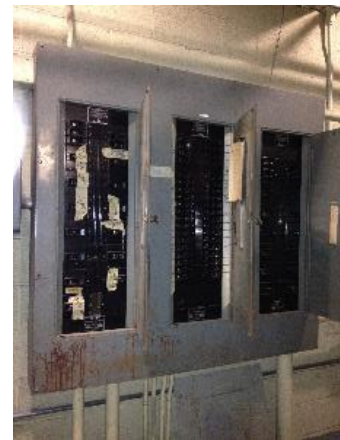
Image 2 – Typical Original FPE Panels
