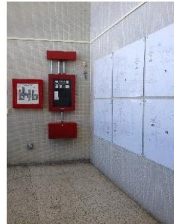
Image 16 – FACP in Main Lobby
