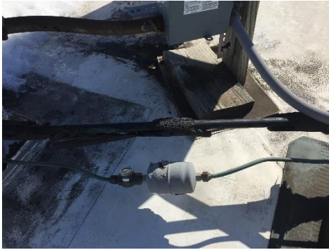
Image 13 – Deteriorated Refrigerant Piping Insulation
