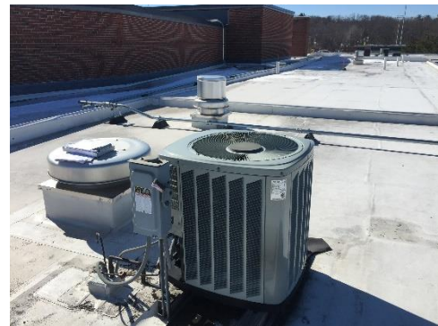
Image 18– Roof Mounted Condensing Unit &amp; Fans
