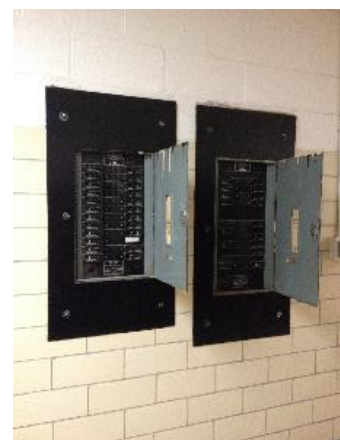
Image 3 – Flush FPE Panels in Corridor
