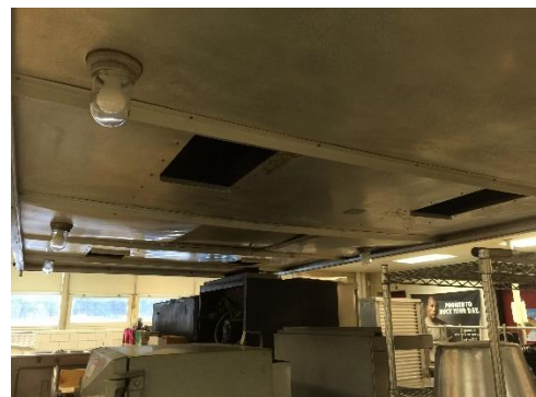
Image 11– Slide Gates Inside Kitchen Hood
