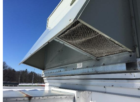
Image 9 – Missing Moisture Elimination Screen on Library RTU
