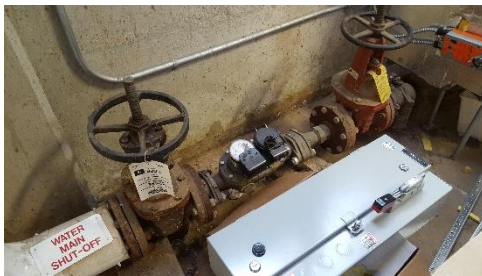
Image 17 – Domestic Water Service & Meter
