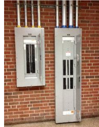
Image 4 – Typical 2005 Panels in Corridor
