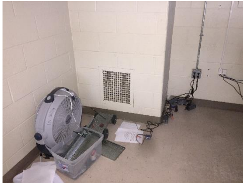
Image 5 – Typical Low Wall Exhaust Grille
