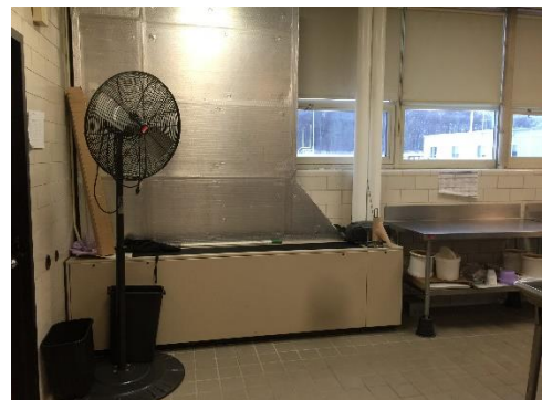
Image 12– Kitchen Unit Ventilator
