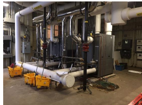
Image 2 - Condensing Boilers (Rear)
