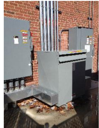
Image 19 –Exterior 300 kVA Step-Down Transformer & Disconnect Switches
