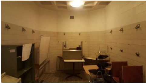
Image 15 – Boys Locker Room Showers
