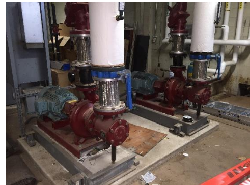
Image 3 - Building Heating Pumps
