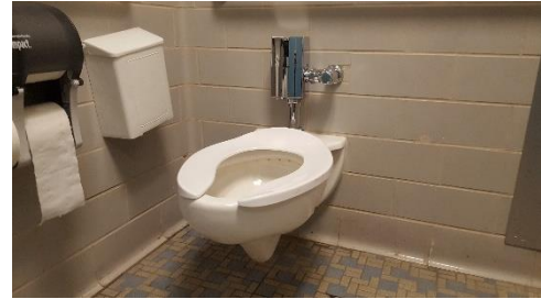
Image 1 – Wall Hung Water Closet
