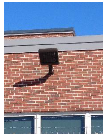
Image 12 – Exterior Wall Fixtures
