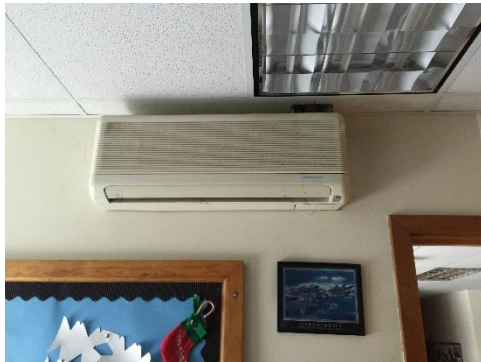
Image 6 – Admin Area Ductless Heat Pump
