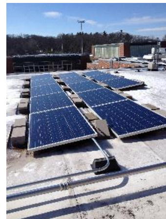
Image 17 – Roof PV Panels
