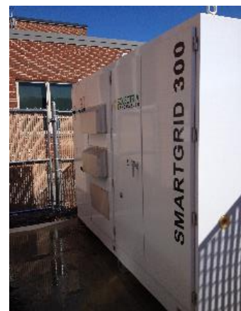
Image 18 – 300 Kw Exterior Inverter
